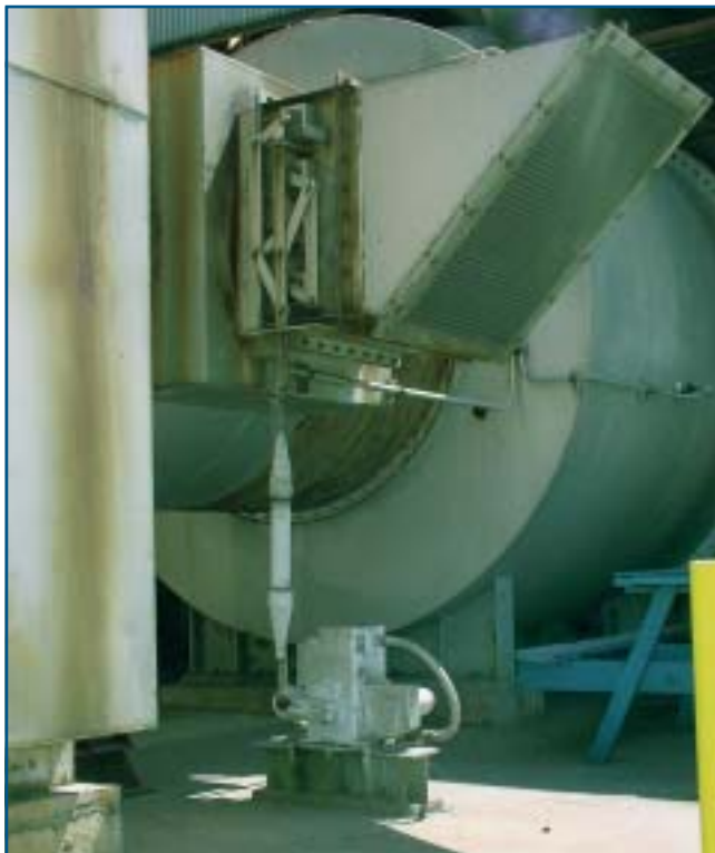
Model 11-200 on a Mixing Air Damper
