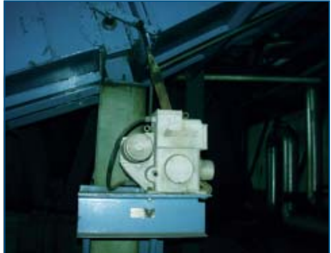
Model 11-400 on an FD Fan Damper
