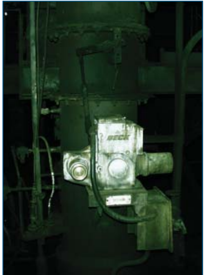
Model 11-200 on an Exhaust Damper
