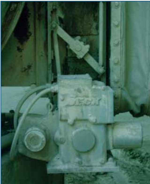
Model 11-200 on a Reverse Air Fan Damper
