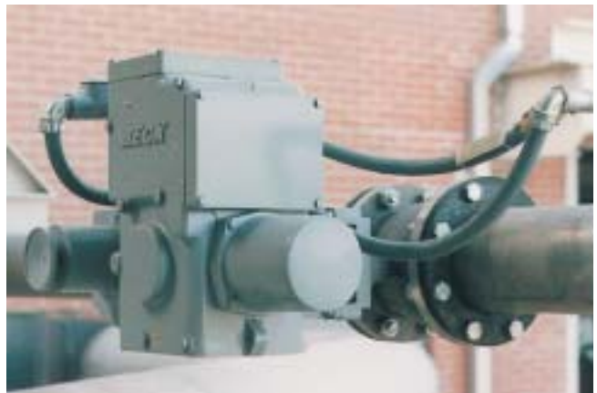
Refiner pressure control valve
