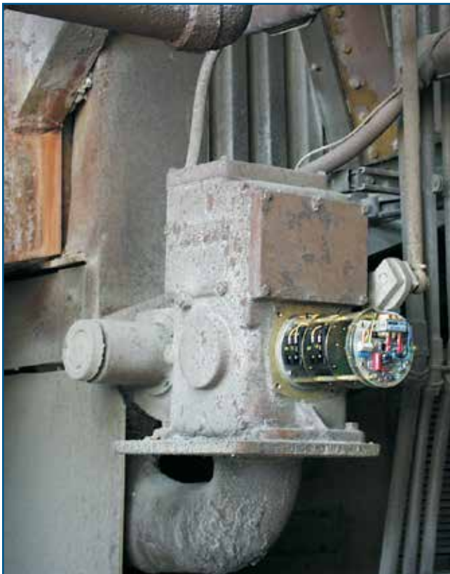
Group 11 actuator with the gasketed control end cover removed
