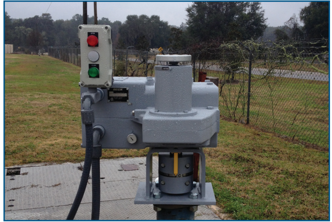
Beck actuator equipped with Remote Indication
