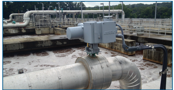
Beck actuator equipped with Remote Indication
