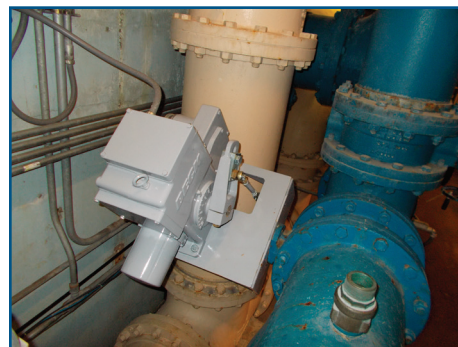
Beck 11-300 actuator mounted on a filter effluent valve.
