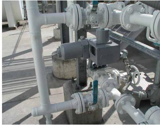
Beck 11E-169 Rotary Valve Actuator on an ethanol/petrol blending application
